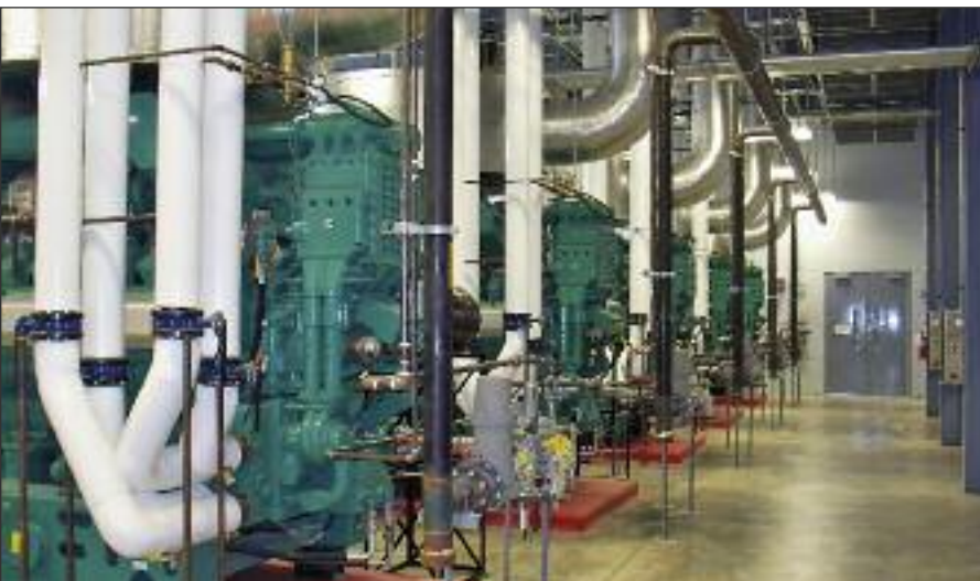
LEFT Five Cummins Power Generation generator sets — four gas and one diesel — installed at a hospital. RIGHT This paralleling switch from Generac Power Systems allows the main power leads of each generator to be connected together at a common point.
